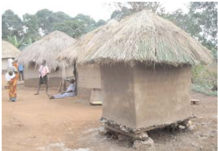
A new granary (Ugandan grain bin) built for storing corn and other grains.
